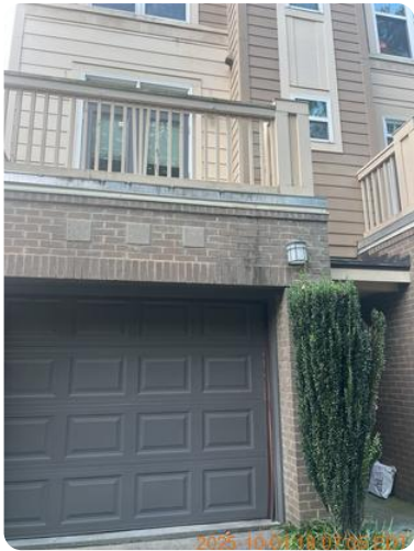
Patio/Deck/Balcony 2025-10-01 18:07:05 35.20553716166199, -80.8161372841898 View Image
