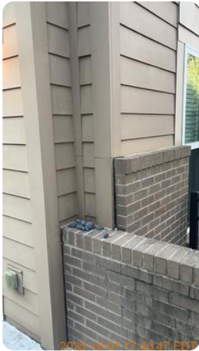
Building Exterior 2025-10-01 17:43:47 35.20526598302308, -80.8161938044133 View Image
