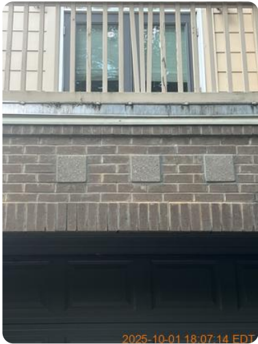
Patio/Deck/Balcony 2025-10-01 18:07:14 35.20553716166199, -80.8161372841898 View Image
