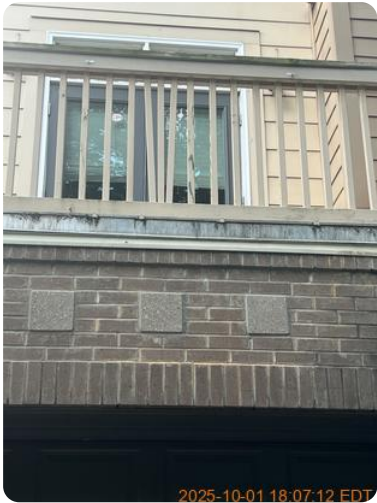
Patio/Deck/Balcony 2025-10-01 18:07:12 35.20553716166199, -80.8161372841898 View Image
