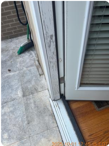
Building Exterior 2025-10-01 17:45:15 35.20526598302308, -80.8161938044133 View Image
