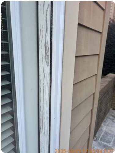
Building Exterior 2025-10-01 17:45:04 35.20526598302308, -80.8161938044133 View Image
