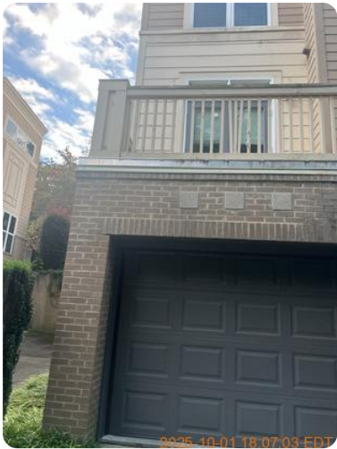
Patio/Deck/Balcony 2025-10-01 18:07:03 35.20045015030755, -80.8154097337165 View Image
